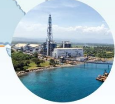
Mindanao Coal Power Plant Phillippines (232 MW e )
