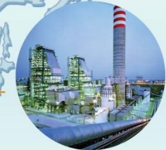
Iskenderun Coal Power Plant Turkey (1,320 MW e )
