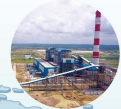
Singareni Coal Power Plant India (1,200 MW e )
