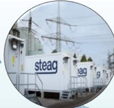
Battery Storage System Germany (90 MW PRL)
