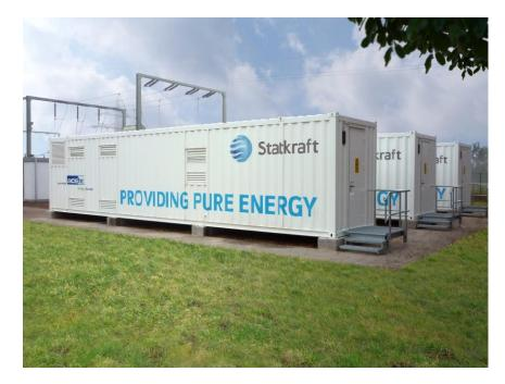
Statkraff's example: 3 batteries in DoerverdenCapacity of one rack:~ 1 MWEnergy storage:~ 1 MWhPrequalified for primary frequency response.
