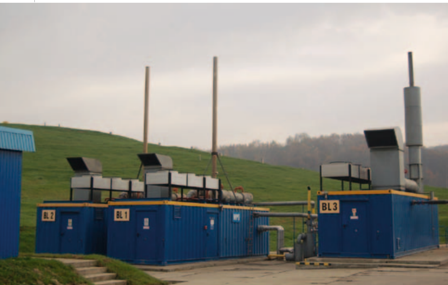
Photo 2. CHP systems in the Barycz landfill near Krakow. Source: a private photo
