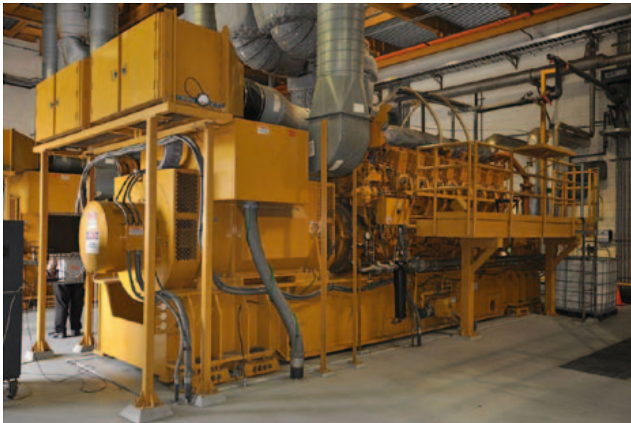
Photo 1. Caterpillar engine powered by landfill gas. Source: a private photo
