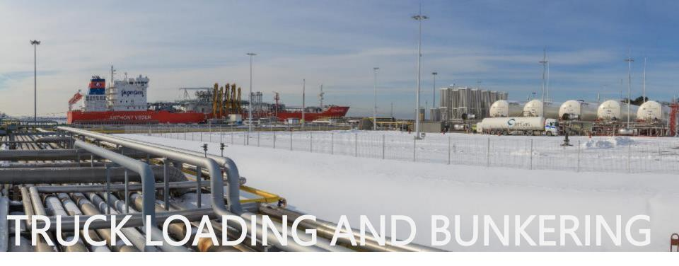
FSRU can be linked (through a pipeline or vessel deliveries) with on-shore tanks to load trucks for off-grid deliveries
