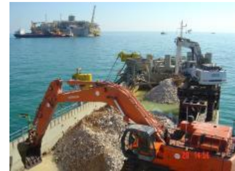
Installation by ballasting and completion
